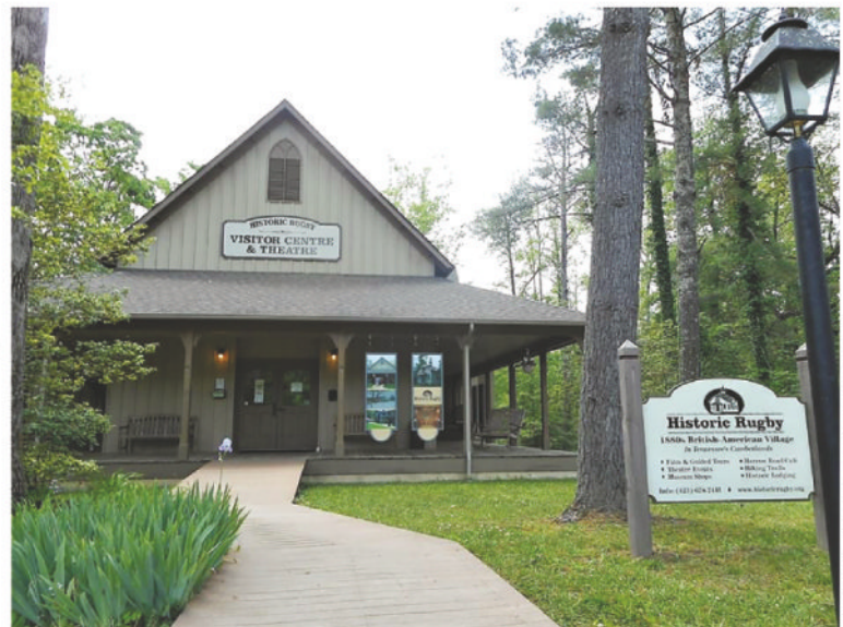
The Visitor Center at Historic Rugby, Tennessee.
