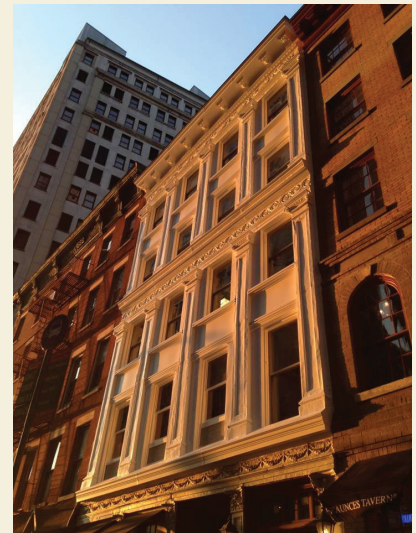
Restored Water Street facade.
