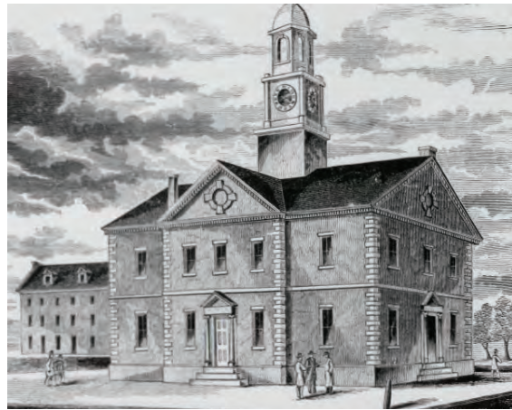
Image of the old Lancaster County Courthouse, where Congress met on 27 Sept 1777.—Source: explorepahistory.com
