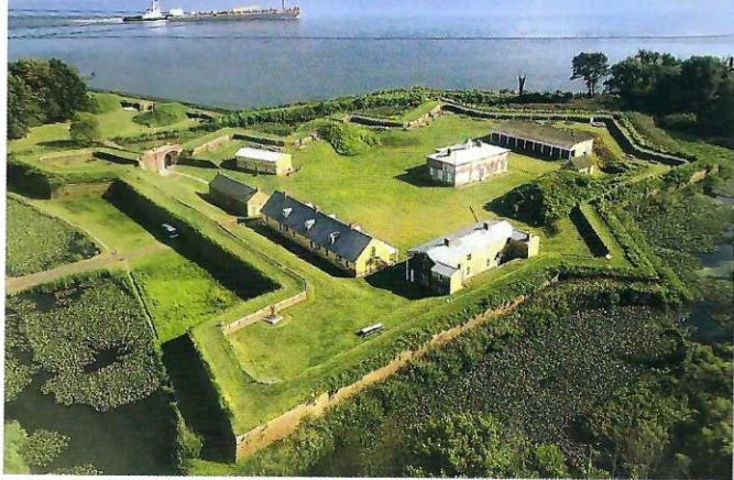
Fort Mifflin, from the air, is a mid-nineteenth century star fort.
